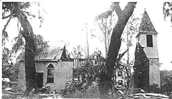
Methodist church after it was hit by a large oak tree and essentially de- stroyed in 1940.
